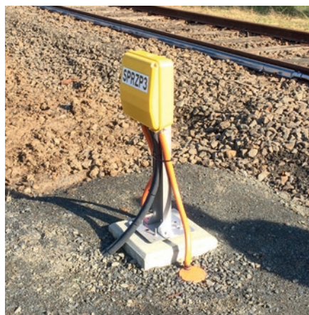
Installed detection point at Stony Point line
