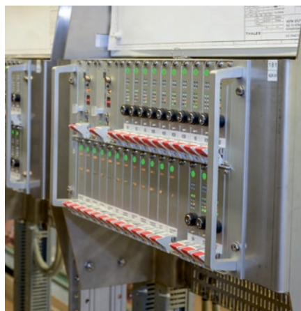
Az LM in Stuttgart's relay interlocking
